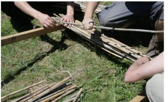
THEN START FIXING BAMBOO CANS TO THE FRAME WITH THE
